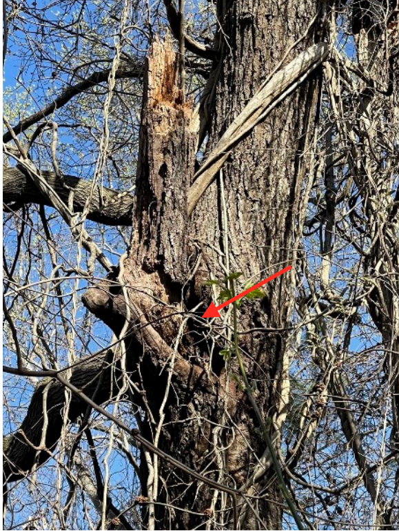
Tree 597 - Vines overtaking canopy; multiple branch failures with decay into main stem
