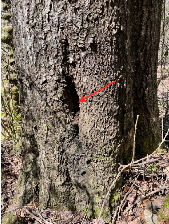
Tree 643 - Small trunk wound opening to larger internal cavity
