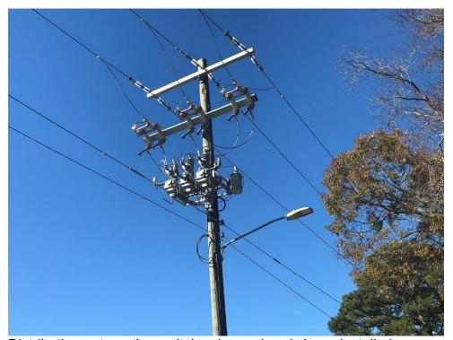
Distribution automation switches have already been installed on Fairway Drive and Herschel Road and will be functional in 2024.
